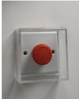
Figure 6. Emergency Electrical shutdown button
